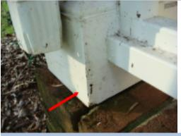
The Column located front porch right side has visible areas of decay at the base. The damage could jeopardize the strength of the column. The decay indicates a history of elevated moisture and or direct water penetration in or around the column area. A licensed general contractor should be consulted for further evaluation, to make necessary repairs, and determine the cause of the deterioration.
