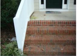
The handrails to the front porch are loose, and present a safety/fall hazard. A licensed general contractor should be consulted for evaluation of the handrail system and to make necessary repairs.
