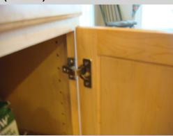
The cabinet hinge was note to be loose/ damaged and in need of repair to ensure proper operation of the cabinet doors. A general repair specialist or licensed general contractor should be consulted for evaluation and repair.
