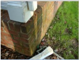
The gutter downspouts are not extended or piped to direct roof drainage away from the foundation. Direct drainage from the gutter system can result in direct water penetration into the foundation area and foundation deterioration. A licensed general contractor should be consulted for a complete evaluation and to make necessary repairs.
