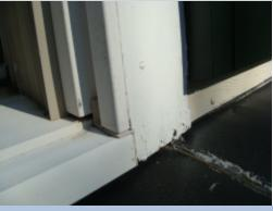
The front bedroom and master bathroom window(s) have soft and decayed wood in the trim area. Decay in the windows can result in leaking and water penetration and should be repaired as soon as possible. All windows should be inspected for similar damage as repairs are made. A licensed general contractor should be consulted to evaluate the extent of the damage and make necessary repairs.
