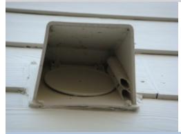
The ventilation fan hood located above rear deck is not operable due to mud dauber tubes. The vent hood needs to be cleaned and inspected to ensure proper operation. A general repair person should be consulted. Owners disclosure is also recommended to identify the fan to which it is connected and proper operation is verified.
