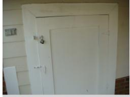
The crawl space door drags and is difficult to open or close. This condition could indicate improper installation or framing movement. The door needs repair/replacement to ensure that the door closes securely and is weather tight. A general repair specialist or licensed general contractor should be consulted for evaluation and repair.
