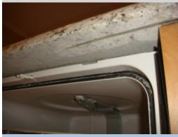
The dishwasher is not secure to the cabinet and it moves forward when the door is opened. The appliance needs to be secured to the cabinet to prevent damage to the unit or personal injury. An appliance repair person or general contractor should be consulted for repair.
