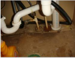
The sink cabinet has visible areas of water damage. The seller should be asked for disclosure related to the damage and history of flooding or leaks. The cabinet needs to be repaired/ replaced and the adjacent plumbing systems evaluated. A general repair specialist should be consulted for evaluation and repair. A licensed plumbing contractor should be consulted for evaluation and repair to ensure proper service.
