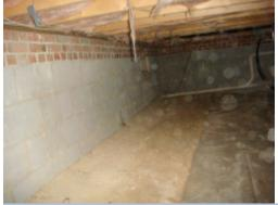
The vapor barrier in the crawl space does not cover the ground completely. Improper installation could result in condensation and inadequate conditioning of the living areas. A licensed general contractor should be consulted for repair/ replacement.
