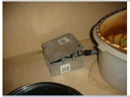
Electrical connections for the counter range top have been made in the cabinet without being properly protected in a covered junction box. The open junction leaves electrical conductors exposed and in a hazardous condition. Electrical concerns should be considered fire and safety issues and repaired as soon as possible. The electrical systems and components in the attic are in need of a complete evaluation and repair by a licensed electrical contractor.
