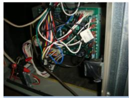
The safety interlock switch located in the attic air handler has been bypassed. The switch is needed to prevent a safety hazards. A HVAC contractor should be consulted to evaluate the system and repair/ replace as needed to ensure proper operation and safe installation.
