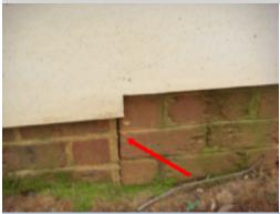
Open cracks were noted in the back porch foundation (left rear) of the home. Cracks in the foundation indicate a deficiency in the foundation, footing, or supporting soil that can change and worsen if it progresses over the life of the home. An engineer should be consulted to determine the significance /cause of the cracks and outline any necessary repairs.
