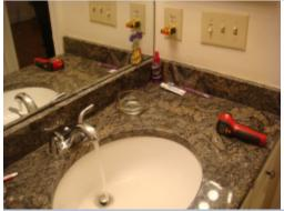
The receptacle had no power. This could indicate a damaged receptacle or branch wiring circuit. A licensed electrical contractor should be consulted for further evaluation and repair.
