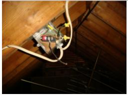
Electrical connections have been made in the top attic area without being properly protected in a covered junction box. The open junction leaves electrical conductors exposed and in a hazardous condition. Electrical concerns should be considered fire and safety issues and repaired as soon as possible. The electrical systems and components in the attic are in need of a complete evaluation and repair by a licensed electrical contractor.
