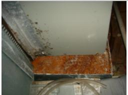
The AC system auxiliary drain pan is in poor condition and in need of replacement. This condition indicates a history of improper drainage of the system condensate water. Improper drainage of the condensate water can result in system and property damage. A HVAC contractor should be consulted for a complete evaluation and to make necessary repairs to ensure safe, reliable, and proper operation of the HVAC system.
