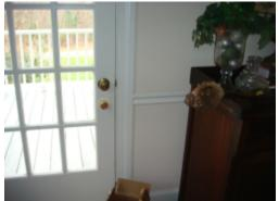
The entrance door to the home has a double key deadbolt lock. This type of lock cannot be unlocked from the interior of the home without the key and is not recommended for main egress doors. In the event of an emergency, the key may not be available resulting in a person not being able to exit the home. Replacement is recommended.
