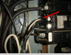
The breaker located on the left side of the electrical panel has two conductors attached to the power screw. Typically breakers are not rated for double taps due to possible loose connections and circuit overloads. This condition presents a safety hazard that could result in interrupted service, property damage, and serious personal injury. A licensed electrical contractor should be consulted for further evaluation and repair.
