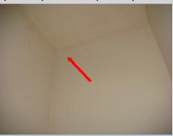
Stains on the ceilings in the right closet indicate a history of a leak. At the time of the inspection it was not possible to determine if the condition was due to an active or past occurrence. Further investigation by a repair specialist and/or owner disclosure is recommended.
