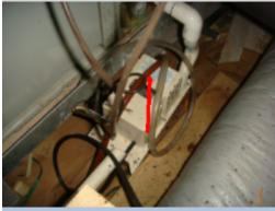
The drainage of the condensate water from the AC system is controlled by a condensate pump. The condensate pump exit drain is contaminated. Improper drainage of the condensate water can result in system and property damage. A HVAC contractor should be consulted for a complete evaluation and repair of the system to ensure safe, reliable, and proper operation of the HVAC system.
