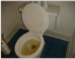
The toilet did not flush completely. The slow flush could be related to a defective flush valve, clogged toilet, or defective toilet. A licensed plumbing contractor should be consulted for evaluation and repair. In addition the door to the toilet room needs repair to ensure proper operation and privacy. The door did not properly close.
