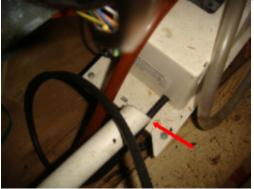
The condensate drain lines are not properly installed with a trap to ensure proper drainage. Improper drainage of the condensate water can result in system and property damage. A HVAC contractor should be consulted for a complete evaluation and repair of the system to ensure reliable and proper operation of the HVAC system.
