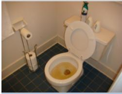
The water in the toilet tanks, sink and tub was noted to be discolored. The discoloration indicates possible defect with the water supply system or distribution piping. The contamination could affect the quality and quantity of the water source for the home. The plumbing supply lines are original to the home. A licensed plumbing contractor should be consulted for complete evaluation of the water supply and distribution systems.
