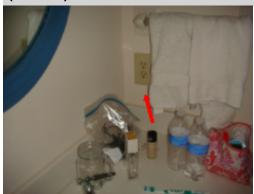
The receptacle(s) located in the master bathroom by sink had no power. This could indicate a damaged receptacle or branch wiring circuit. A licensed electrical contractor should be consulted for further evaluation and repair.
