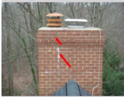
The mortar is deteriorated and cracked. When the mortar cap is damaged water can enter between the chimney body and the flue liner resulting in leaks and deterioration. A masonry contractor should be consulted for a complete evaluation of the chimney, the flue liner and the masonry crown and to make necessary repairs.
