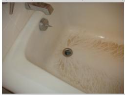
The linkage for the tub drainage stopper is not functioning properly. The stopper needs repair to ensure that the tub can be filled and easily drained. A licensed plumber should be consulted for repair.
