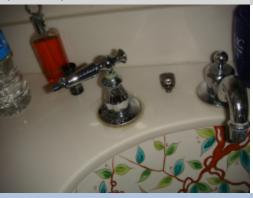
The sink faucet left sink hot faucet leaks at the handle base area when turned on. The leaks could result in damage to the sink and cabinet and should be repaired as soon as possible. A licensed plumbing contractor should be consulted for a complete evaluation to determine the significance of this concern and make necessary repairs to prevent leaks and ensure sanitary conditions.
