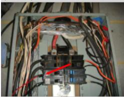
Several breakers in the electrical panel has two conductors attached to the power screw. Typically breakers are not rated for double taps due to possible loose connections and circuit overloads. This condition presents a safety hazard that could result in interrupted service, property damage, and serious personal injury. A licensed electrical contractor should be consulted for further evaluation and repair.
