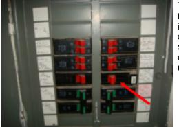
The breaker labeled for bathrooms in the panel was noted to be in the tripped position at the time of the inspection. A tripped breaker indicates a problem with the branch circuit or the appliance. This condition presents a safety hazard that could result in interrupted service, property damage, and serious personal injury. A licensed electrical contractor should be consulted for further evaluation and repair.
