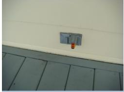
The receptacle(s) located front balcony had no power. This could indicate a damaged receptacle or branch wiring circuit. A licensed electrical contractor should be consulted for a complete evaluation to determine the significance of this concern and make necessary repairs to correct defects and prevent safety hazards.
