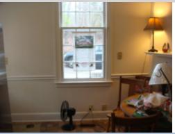
The window in the kitchen needs repair to ensure proper operation. The window could not be opened. A licensed general contractor should be consulted for evaluation and repair.
