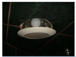
The light fixture located in the shower is not a sealed unit. The light fixture should be verified to be rated for installation in a wet environment. A licensed electrical contractor should be consulted for evaluation and repair to ensure safe and proper service.
