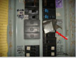
The electrical service panel cover is missing knock out opening plugs. The covers or plugs prevent direct contact with hot electrical circuits. This condition presents a safety hazard that could result in interrupted service and serious personal injury /death from electrocution. A licensed electrical contractor should be consulted for a complete inspection of the electrical system and for repair/replacement of the panel to ensure that it is safe and functioning properly.
