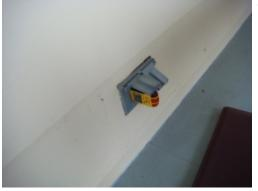
The receptacle(s) located on rear balcony had no power. This could indicate a damaged receptacle or branch wiring circuit. A licensed electrical contractor should be consulted for a complete evaluation to determine the significance of this concern and make necessary repairs to correct defects and prevent safety hazards.
