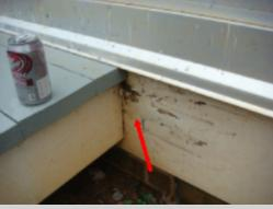
The exterior steps going onto the rear enclosed porch have areas of decay. A licensed general contractor should be consulted for a complete evaluation of the exterior of the home to determine the extent of the damage to the siding, trim, and underlying components to ensure the weathertightness of the system.
