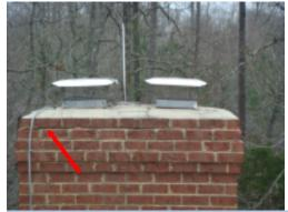
The mortar is deteriorated and cracked. When the mortar cap is damaged water can enter between the chimney body and the flue liner resulting in leaks and deterioration. A masonry contractor should be consulted for a complete evaluation of the chimney, the flue liner and the masonry crown and to make necessary repairs.
