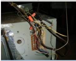
The attic air handler electrical systems and components in the attic are in need of a complete evaluation and repair by a licensed electrical contractor. The following electrical concerns were noted: Junction Boxes no cover; Junctions no boxes; Service cables not supported.
