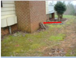
The cleanout door is damaged and in need of repair/replacement. A chimney sweep and general contractors should be consulted for a complete evaluation of the chimney and to make necessary repairs to ensure that the chimney is safe and functional.
