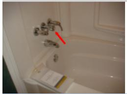
The shower/ diverter valve did not function properly. A licensed plumbing contractor should be consulted for evaluation and repair to ensure proper service.
