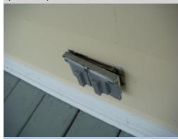
The receptacle located on front porch right is loose. Loose receptacles could result in electrical shock hazard or property damage. A licensed electrical contractor should be consulted for a complete evaluation to determine the significance of this concern and make necessary repairs to correct defects and prevent safety hazards.
