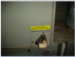
The condensate drain lines are not properly installed with a trap to ensure proper drainage. Improper drainage of the condensate water can result in system and property damage. A HVAC contractor should be consulted for a complete evaluation and repair of the system to ensure reliable and proper operation of the HVAC system.
