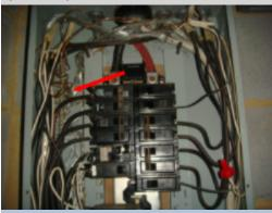
The neutral bus bar located on the left side of the panel is not isolated from the ground system. This condition presents a safety hazard that could result in interrupted service, property damage, and serious personal injury. A licensed electrical contractor should be consulted for repair and a complete evaluation of the electrical system.
