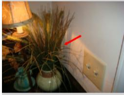
The receptacle located first floor bathroom is not GFCI protected. Receptacles located in hazardous or wet locations should be GFCI protected to reduce shock in hazardous locations. A licensed electrical contractor should be consulted for further evaluation and repair.
