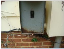
Evidence suggests that water has been entering the main electrical service panel. This condition presents a safety hazard that could result in interrupted service, property damage, and serious personal injury. The panel cover was not removed and the inspection was not completed. A licensed electrical contractor should be consulted for a complete inspection of the electrical system and for repair/replacement of the panel to ensure that it is safe and functioning properly.
