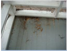
The wood deck was found to be in poor condition. Areas of soft wood were discovered. A licensed general contractor should be consulted for complete evaluation of the deck and to make necessary repairs or replacement as needed.
