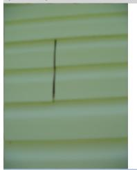
on the rear of the house, short pieces of siding were noted. The short pieces are loose and leave the wall sheathing/house wrap exposed. The siding needs to be installed to create a complete cladding system covering all underlying wall components. A siding installation company or general contractor should be consulted to evaluate and repair the siding to ensure the integrity of the cladding system.
