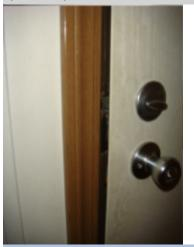
The door lock assembly is not aligned with the striker in the jamb area. The deadbolt could not be engaged to secure the door. The door/lock needs repair/replacement to ensure that the door closes securely. A general repair specialist or licensed general contractor should be consulted for evaluation and repair.
