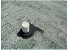
The vent boot located left and middle of roof acts as a flashing to prevent water penetration around the plumbing vent pipe is split, cracked. A licensed roofing contractor should be consulted for evaluation and repair to ensure the weather-tightness of the roof covering system.
