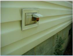
The receptacle located main house rear had no power. This could indicate a damaged receptacle or branch wiring circuit. A licensed electrical contractor should be consulted for a complete evaluation to determine the significance of this concern and make necessary repairs to correct defects and prevent safety hazards.
