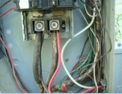
A set of conductors for the external generator plug have been inserted in the main lugs with the main service cables. This double tap leaves the added conductors and branch circuit that is being power unprotected and unsafe. This condition presents a safety hazard that could result in interrupted service, property damage, and serious personal injury. A licensed electrical contractor should be consulted for repair and a complete evaluation of the electrical system.
