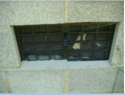
The foundation vents on right side of house are not operating properly. Improper ventilation could result in condensation and elevated moisture levels in building components. A licensed general contractor should be consulted for a complete evaluation of the crawl space to determine the significance of the concern and make necessary repairs. Refer to the foundation section of the report.
