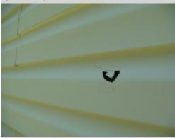
On the left side of the home, a damaged or cracked piece of siding is in need of replacement. A siding installation company or general contractor should be consulted to evaluate and repair the siding to ensure the integrity of the cladding system.
