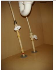
The sink faucet leaks into the cabinet area when turned on. The leaks could result in damage to the sink and cabinet and should be repaired as soon as possible. A licensed plumbing contractor should be consulted for a complete evaluation to determine the significance of this concern and make necessary repairs to prevent leaks and ensure sanitary conditions.
