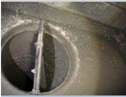
From the fireplace opening, heavy build of soot was noted. Soot build-up can result in improper function of the fireplace and high potential for fire. A chimney sweep and general contractors should be consulted for a complete evaluation of the chimney and to make necessary repairs to ensure that the chimney is safe and functional.
