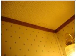
Stains on the ceilings indicate a history of a leak. At the time of the inspection it was not possible to determine if the condition was due to an active or past occurrence. Further investigation by a repair specialist and owner disclosure is recommended.
