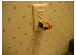
The receptacle located in bathroom #1 had no power. This could indicate a damaged receptacle or branch wiring circuit. A licensed electrical contractor should be consulted for a complete evaluation to determine the significance of this concern and make necessary repairs to correct defects and prevent safety hazards.
