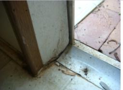
The exterior rear door trim has soft and decayed wood in the frame area bottom left. Decay in the door frames can result in leaking and water penetration and should be repaired as soon as possible. All doors should be inspected for similar damage as repairs are made. A general repair specialist or licensed general contractor should be consulted for evaluation and repair.
