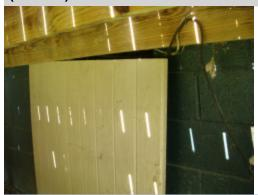
Access to the crawl space under the back deck is not secure, and can allow unwanted animals access. A general contractor should be consulted for further evaluation and to make necessary repairs.
