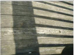
The deck surface boards are cupped and splintered. Splintering boards can result in injury such as puncture wounds and should be considered hazardous for children. A licensed general contractor should be consulted for evaluation and to make necessary repairs.
