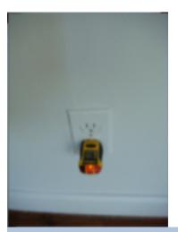
The receptacles located in various rooms throughout the house tested as open ground, even though receptacles are three prongs. An equipment ground provides an extra safety feature to prevent electrical shock hazards and property damage. A licensed electrical contractor should be consulted for a complete evaluation to determine the significance of this concern and make necessary repairs to correct defects and prevent safety hazards.
