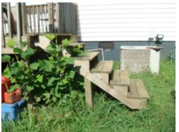
The deck steps do not have handrails to prevent accidentally falling or stepping off the floor surface. It is recommended that handrails be installed to ensure safe and functional use of the deck. A licensed general contractor should be consulted for a complete evaluation and to make necessary repairs.
