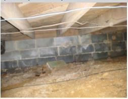
Insulation and vapor barrier in the crawl space is missing. Improper insulation installation could result in condensation, over heating of the building components, and inadequate conditioning of the living areas. A licensed general contractor should be consulted for repair/replacement.
