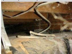
Disconnected wires were noted in the crawl space. Disconnected wires should be removed or properly terminated. The disconnected wires leave electrical conductors exposed and in a hazardous condition. Electrical concerns should be considered fire and safety issues and repaired as soon as possible. The electrical systems and components are in need of a complete evaluation and repair by a licensed electrical contractor.
