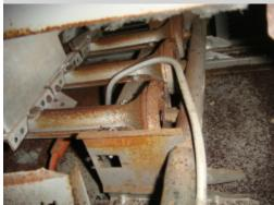
The gas furnace unit has visible rust in the burner chamber area. The rust indicates deterioration of the exchanger. Deterioration of the heat exchanger is a serious concern that can result in improper combustion and carbon monoxide poisoning. The furnace needs a complete evaluation which should include a heat exchanger inspection to ensure safe, reliable, and proper operation of the HVAC system. A licensed HVAC contractor should be consulted for repair.
