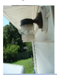
The light fixture located on the rear deck was not functional when tested. This could indicate a defective bulb or other more serious problem such as faulty wiring or a defective fixture, further evaluation and repair is needed. A licensed electrical contractor should be consulted for further evaluation and repair.
