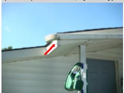
The gutter trays and downspouts in various locations around the house are loose and not properly secured. Loose gutter trays can be the result of physical damage or improper support spacing. It is very important to keep gutter functioning properly to reduce direct drainage to the foundation and wall cladding systems. A licensed general contractor should be consulted for a complete evaluation and to make necessary repairs.
