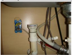
An electrical receptacle was noted in the cabinet behind the storage. The receptacle is missing the cover plate. Exposed uncovered receptacles and junction boxes are fire hazards. A licensed electrical contractor should be consulted for a complete evaluation to determine the significance of this concern and make necessary repairs to correct and prevent safety hazards.
