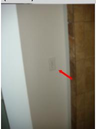
The receptacles located in both bathrooms are not GFCI protected. Receptacles located in hazardous or wet locations should be GFCI protected to reduce shock in hazardous locations. A licensed electrical contractor should be consulted for further evaluation and repair.
