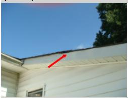
The additions roof slopes to one side and the roof sheathing edges are not supported parallel to the rafter in the roof valley area. The edges of the roof sheathing need to be supported along the long seams parallel to the rafters and beams to prevent movement and damage to the roof covering. A licensed general contractor should be consulted for further evaluation and to make necessary repairs.
