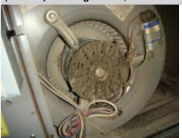
The air handler cabinet is dirty and in poor condition. The condition of the cabinet ensures protection of the coil/fan and clean air supply. A HVAC contractor should be consulted for a complete evaluation and to make necessary repairs to ensure safe, reliable, and proper operation of the HVAC system.
