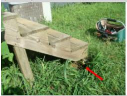
The wood steps for the rear deck are in need of repair. The steps should be repaired to ensure safe entry and egress for the home. The following concerns were noted at the time of the inspection: Step stringer base is not properly supported; A licensed general contractor should be consulted for a complete evaluation and to make necessary repairs.
