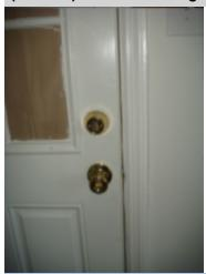
The entrance door to the home has a double key deadbolt lock. This type of lock cannot be unlocked from the interior of the home without the key and is not recommended for main egress doors. In the event of an emergency, the key may not be available resulting in a person not being able to exit the home. Replacement is recommended.
