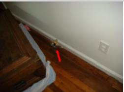
This home has corrugated stainless steel gas lines. This gas line has specific installation requirements related to required bending allowances, support, protection, and electrical bonding to ensure safe conditions. A section of the CSST gas line located in main hallway is not in use and should have a permanent sealing cap installed.
