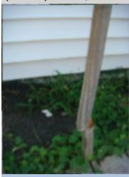
Incorrect baluster spacing and several balusters were noted to be loose or damaged and in need of repair or replacement to ensure safe and functional use of the deck/porch. A licensed general contractor should be consulted for a complete evaluation and to make necessary repairs.
