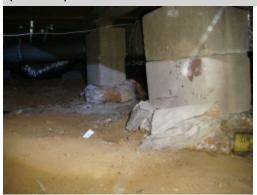
The foundation and pier system are in need of repair. This foundation was constructed without a concrete footing, over time the soil under the foundation area has eroded and degraded leaving the foundation poorly supported. A licensed general contractor should be consulted for further evaluation and repair. If the repair is beyond the scope of the Building code, a professional engineer should be consulted to outline the repair.
