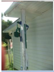
The column is weathered and starting to split. Repair and painting is needed to prevent further damage and decay. A general repair person should be consulted.
