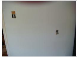
The receptacle is missing the cover plate. Exposed uncovered receptacles and junction boxes are fire hazards. A licensed electrical contractor should be consulted for a complete evaluation to determine the significance of this concern and make necessary repairs to correct and prevent safety hazards.
