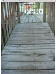
The front porch surface boards are cupped and splintered. Splintering boards can result in injury such as puncture wounds and should be considered hazardous for children. A licensed general contractor should be consulted for evaluation and to make necessary repairs.
