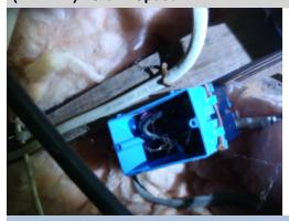
Electrical connections have been made in the crawl space without being properly protected in a covered junction box. The damage leaves electrical conductors exposed and in a hazardous condition. Electrical concerns should be considered fire and safety issues and repaired as soon as possible. The electrical systems and components are in need of a complete evaluation and repair by a licensed electrical contractor.
