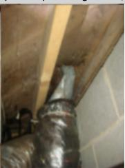
The insulation for the duct branches is not fully insulated to the registers. The insulation prevents condensation from building and causing the floor to deteriorate at the register. A HVAC contractor should be consulted for a complete evaluation and replacement of all damaged duct components to ensure reliable and proper operation of the HVAC system.
