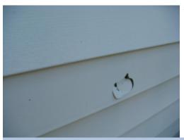
The siding for this home is a vinyl material. The siding on this home has several visible areas of damaged pieces. A licensed general contractor should be consulted for complete evaluation to locate and repair all areas of damage.
