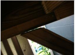
The deck bracing was loose. Loose bracing can cause lateral movement of the deck. Improper deck construction can result in unsafe conditions and possible deck failure. A licensed general contractor should be consulted for complete evaluation of the deck and to make necessary repairs.
