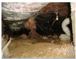
The insulation on the duct trunk line was noted to be wet. The source of the moisture and any related concerns need to be addressed to ensure proper air flow and prevent contamination of the air supply. A HVAC contractor should be consulted for a complete evaluation and replacement of all damaged duct components to ensure reliable and proper operation of the HVAC system.
