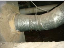
The gas furnace has a natural draft exhaust system. The flue exits directly to the side wall without the require height of vertical rise. This configuration creates a hazard that could result in exhaust entering the living spaces of the home and possible carbon monoxide poisoning. A HVAC contractor should be consulted for a complete evaluation and repair of the system to ensure safe and proper operation of the HVAC system.
