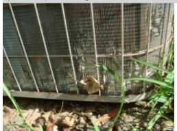
The outside compressor/coil unit for the AC system has visible damage to the coil fins. A damaged coil can result in leaking refrigerant and poor system performance. A HVAC contractor should be consulted for a complete evaluation and repair of the system to ensure reliable and proper operation of the HVAC system.
