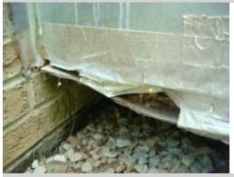
The insulation cover for the duct branch that supplies first floor is deteriorated. The cover protects the duct structure and holds the insulation in place. A HVAC contractor should be consulted for a complete evaluation and replacement of all damaged duct components to ensure reliable and proper operation of the HVAC system.
