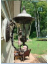
The light fixture located by right side door was not functional when tested. This could indicate a defective bulb or other more serious problem such as faulty wiring or a defective fixture, further evaluation and repair is needed. A licensed electrical contractor should be consulted for further evaluation and repair.
