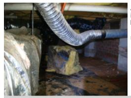
A section of insulation in the crawl space is missing. Improper insulation installation could result in condensation, over heating of the building components, and inadequate conditioning of the living areas. A licensed general contractor should be consulted for repair/ replacement.
