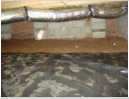
The vapor barrier for the crawl space insulation was not covering all areas. Improper installation could result in condensation, A licensed general contractor should be consulted for repair/ replacement.
