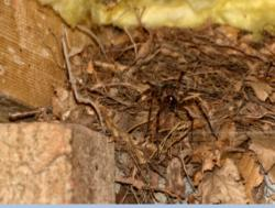
spiders and nest were noted in the crawl space. While not uncommon, pests can cause damage to building components and unsanitary/ unsafe conditions. A general contractor or pest management company should be consulted to locate and correct the points of entry and determine the extent of the contamination.
