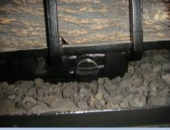
The gas log fireplace located in the living room was visually inspected but not operated because the pilot was off. The unit should be serviced and operated prior to closing to ensure safe and proper operation of the HVAC system.
