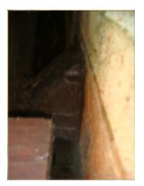
The exit for the dryer exhaust is restricted. This can result in trapped lint and create a fire hazard. A licensed general contractor or general repair specialist should be consulted for further evaluation to make sure the duct is properly installed, not clogged, and to make necessary repairs.
