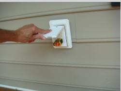
The receptacle located porch right side had no power. This could indicate a damaged receptacle or branch wiring circuit. A licensed electrical contractor should be consulted for a complete evaluation to determine the significance of this concern and make necessary repairs to correct defects and prevent safety hazards.
