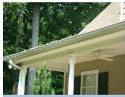
The gutter on both front and rear of house are filled with debris. Direct drainage from the gutter system can result in water penetration into the foundation area and foundation deterioration. A licensed general contractor should be consulted for a complete evaluation and to make necessary repairs.
