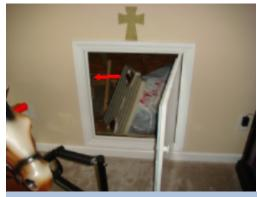
The light fixture located in the attic access at top landing of stairs was not functional. This could indicate a defective bulb or unable to find correct switch or other more serious problem such as faulty wiring or a defective fixture, further evaluation and repair is needed. A licensed electrical contractor should be consulted for further evaluation and repair.
