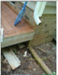
The gutter downspouts are not extended or piped to direct roof drainage away from the foundation. Direct drainage from the gutter system can result in direct water penetration into the foundation area and foundation deterioration. A licensed general contractor should be consulted for a complete evaluation and to make necessary repairs.
