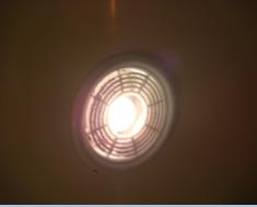
The ventilation fan is clogged and did not operate properly. The fan needs repair/ replacement to ensure proper ventilation and moisture control. A general repair specialist should be consulted.
