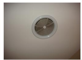
The ventilation fan has lint in the grill area and on the exterior exit at the roof surface. The fans needs to be cleaned and inspected to ensure proper operation. A general repair person should be consulted.
