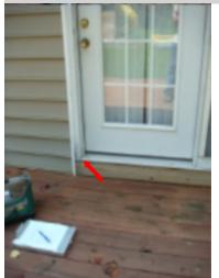
The door has the beginnings of decayed wood in the frame area. Decay in the door frames can result in leaking and water penetration and should be repaired as soon as possible. All doors should be inspected for similar damage as repairs are made. A general repair specialist or licensed general contractor should be consulted for evaluation and repair.
