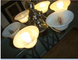
The light fixture located in the dinning room was not fully functional when tested. This could indicate a defective bulb or other more serious problem such as faulty wiring or a defective fixture, further evaluation and repair is needed. A licensed electrical contractor should be consulted for further evaluation and repair.
