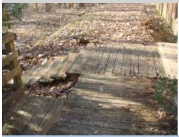
The wood deck walk/ steps in the left rear was found to be in poor condition. A licensed general contractor should be consulted for complete evaluation of the deck and to make necessary repairs or replacement as needed.
