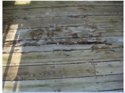
Some of the deck surface boards are cupped, splintered decayed. Splintering boards can result in injury such as puncture wounds and should be considered hazardous for children. A licensed general contractor should be consulted for evaluation and to make necessary repairs.
