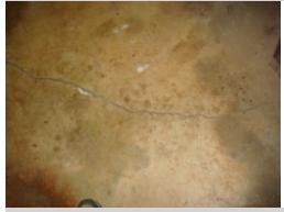
The basement floor pad is cracked. The pad surface was even and no evidence of differential movement was noted. A general repair person should be consulted to seal the crack to prevent water penetration.
