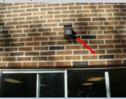
The light fixture located out side sliding basement door was not functional when tested. This could indicate a defective bulb or other more serious problem such as faulty wiring or a defective fixture, further evaluation and repair is needed. A licensed electrical contractor should be consulted for further evaluation and repair.
