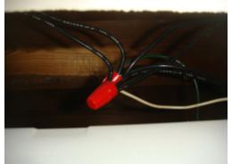
Electrical connections have been made in the finished basement area above the dropped ceiling without being properly protected in a covered junction box. The open junction leaves electrical conductors exposed and in a hazardous condition. Electrical concerns should be considered fire and safety issues and repaired as soon as possible. The electrical systems and components in the attic are in need of a complete evaluation and repair by a licensed electrical contractor.
