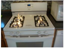
The top burners for the range did not function properly. Flames were yellow and uneven, improper burners can result in improper operation and dangerous level of carbon monoxide in the appliance exhaust. An appliance repair person should be consulted for further evaluation and repair to ensure safe and proper operation of the appliance.
