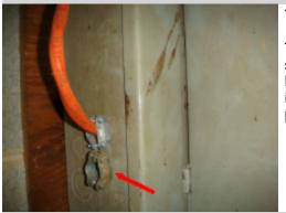
The electrical service panel cover is missing knock out opening plugs. The covers or plugs prevent direct contact with hot electrical circuits. This condition presents a safety hazard that could result in interrupted service and serious personal injury /death from electrocution. A licensed electrical contractor should be consulted for a complete inspection of the electrical system and for repair/replacement of the panel to ensure that it is safe and functioning properly.
