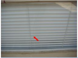
The right front bedroom window needs further evaluation and repair. The window was cracked. All windows should be evaluated as repairs are made. A licensed general contractor should be consulted. Refer to the exterior section of the report.
