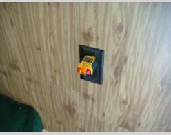
Two receptacle(s) located finished part of the basement tested as reversed polarity. Polarization provides an extra safety feature to prevent electrical shock hazards and property damage. A licensed electrical contractor should be consulted for a complete evaluation to determine the significance of this concern and make necessary repairs to correct defects and prevent safety hazards.
