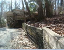
The front section of the lot for this home is a steep grade that is currently retained by a wood timber wall. Retaining this section of the lot will be very important over the life of this home. An engineer should be consulted for a complete inspection of the retaining system prior to purchase.
