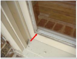
Window glazing is installed in the window frame to secure the glass panes. The glazing on many of the windows for this home is loose, cracking and missing. The windows need repairs and painting to secure window panes, prevent decay and leaking. A licensed general contractor should be consulted to make necessary repairs.
