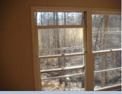
Many window throughout the house are either hard to open or the top will not stay in position. and need repair to ensure proper operation. In the case of bedroom windows It is very important to have a proper method of egress from every sleeping area in case of an emergency such as a fire. A licensed general contractor should be consulted for evaluation and repair.
