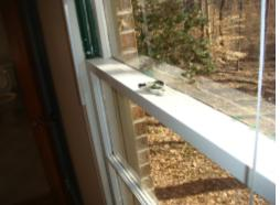
The window for the master bedroom needs repair to ensure proper operation. The window did not properly lock. All windows should be evaluated as repairs are made. A licensed general contractor should be consulted.
