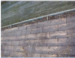
The gutter in the front of the house is clogged. Clogged gutters can lead to unwanted water penetration . A licensed general contractor should be consulted to make necessary repairs.
