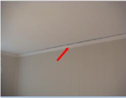
In the dinning room, and hallway The junction of the wall and ceiling has a gap. No related concerns were noted throughout the adjacent inspection areas. The buyer should review the area of concern. If additional concerns or questions are present, invasive inspection and repair will be needed. A general repair specialist should be consulted for evaluation and repair.
