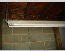
The light fixture located in the unfinished basement was not functional when tested. This could indicate a defective bulb or other more serious problem such as faulty wiring or a defective fixture, further evaluation and repair is needed. A licensed electrical contractor should be consulted for further evaluation and repair.
