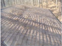
The shingles for the home are covered with a heavy build- up of leaves/pine needles/debris. This limited the inspection of the roof surface. Debris on the roof surface can trap moisture allow water and debris to travel under the shingle tabs resulting in material failure and leaks. A roofing contractor should be consulted to remove the debris and inspect the shingles / adjacent component for evidence of damage and make necessary repairs.
