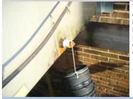
The condensate drain lines are not properly attached to the inside coil. The drain lines are attached to the line openings provided for horizontal / vertical installation and the unit is installed in the vertical / horizontal location. Improper drainage of the condensate water can result in system and property damage. A HVAC contractor should be consulted for a complete evaluation and repair of the system to ensure reliable and proper operation of the HVAC system.
