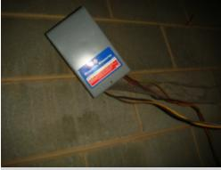
The electrical panel is not secure where it is attached to the wall of the home. This condition presents a safety hazard that could result in serious personal injury and or property damage. The electrical panel cover was not removed and the inspection was not completed. A licensed electrical contractor should be consulted for a complete inspection of the electrical system and for repair/replacement of the panel to ensure that it is safe and functioning properly.
