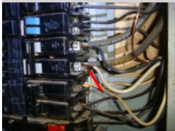
Two breakers located on the right side of the electrical panel has two conductors attached to the power screw. Typically breakers are not rated for double taps due to possible loose connections and circuit overloads. This condition presents a safety hazard that could result in interrupted service, property damage, and serious personal injury. A licensed electrical contractor should be consulted for further evaluation and repair.
