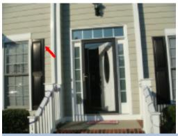
The window shutter was noted to be loose. If the shutter is not properly installed it will not prevent water penetration. A siding installation company or general contractor should be consulted to evaluate and repair the siding to ensure the integrity of the cladding system.
