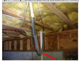
The drainage pipe from the dishwasher to the sink plumbing was not installed in manner to prevent sewer from backing up in the event of a plumbing clog. The dishwasher needs further evaluation and repair to ensure sanitary and proper operation. An appliance repair person should be consulted.
