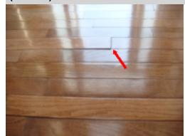
In the front hallway a hardwood floor board was raised. Excessive movement of the hardwood floors can indicate improper installation and or unbalanced moisture conditions that indicate underlying problems. A flooring installation/ repair company should be consulted for further evaluation to determine the significance and source of the concern.
