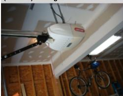
The garage door needs adjustment and repair. The door did not stop/reverse when the path was interrupted. A garage door installation company or a licensed general contractor should be consulted for evaluation and repair to ensure that the door operates safely and properly.
