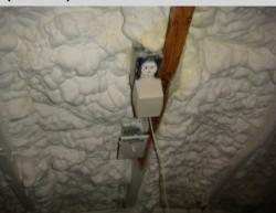
The receptacle located attic is missing cover plate. Missing cover plates could result in increased shock and fire hazards. A licensed electrical contractor should be consulted to make necessary repairs to ensure safe and proper operation and installation.
